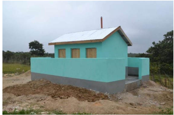
Completed new toilet block at Mariani Primary School
